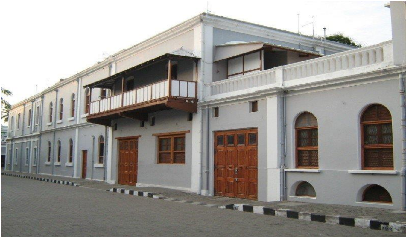
Back side view of Sri Aurobindo Ashram – Puducherry
